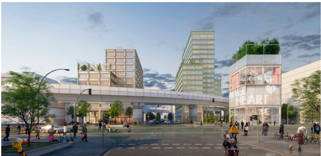
View into town from Nordkanalstraße: The S-Bahn viaduct runs through the new complex. A staggered group of buildings (middle) offers modern working environments right at the bend of the S-Bahn line.
