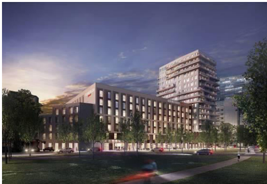
Once completed, "KONRAD" will enrich the Hamburg's skyline with its 60-metre-high tower.
